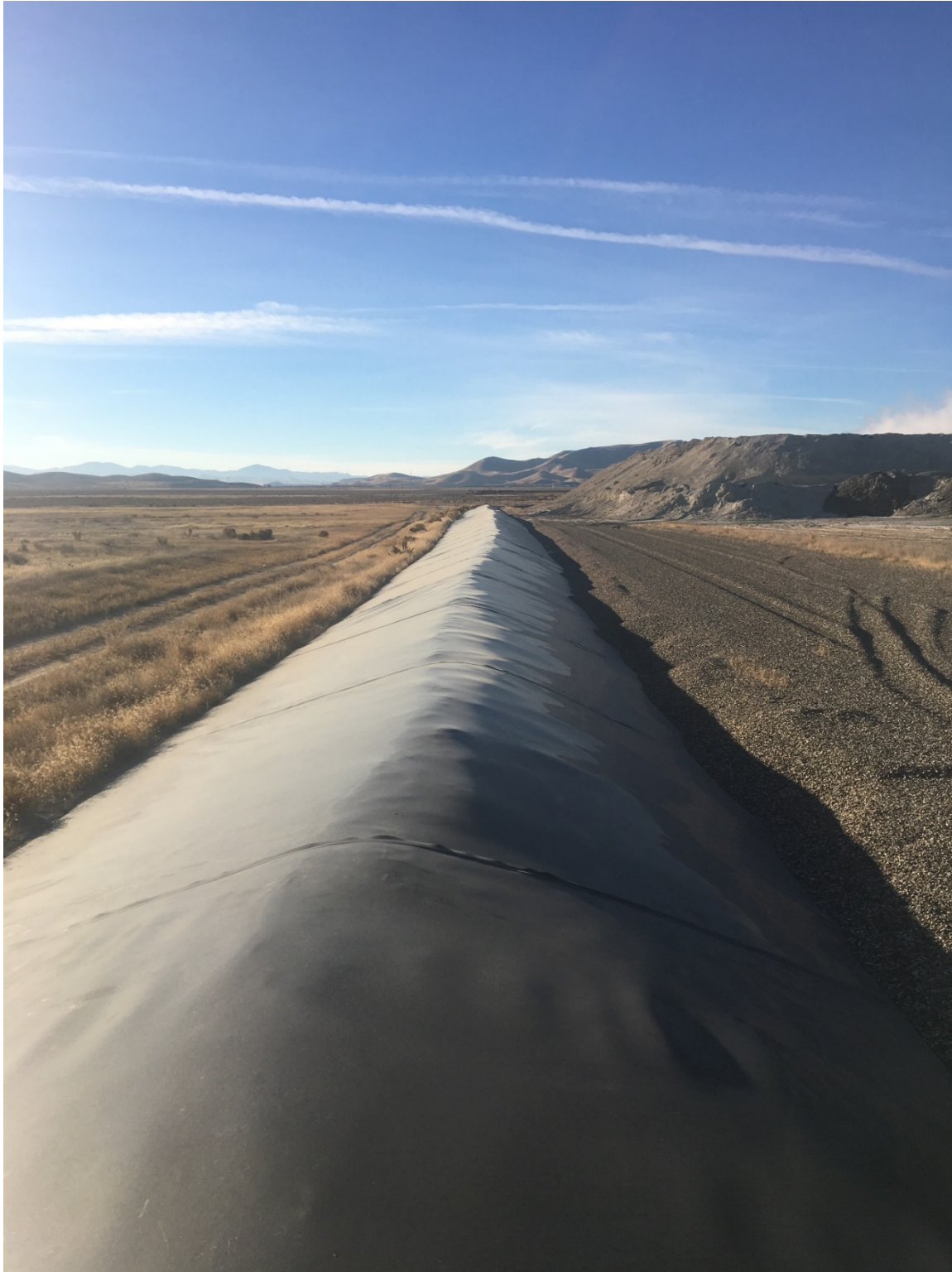
Photo 7. East Perimeter Berm, Northeast Corner, Cell 1 and 2 - View South
