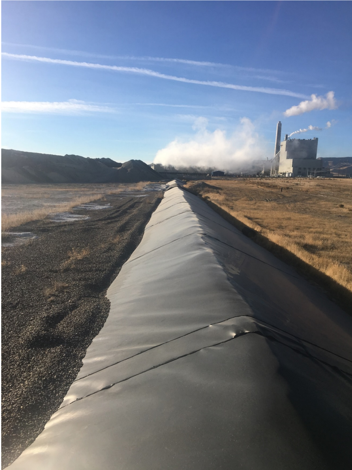
Photo 11. West Perimeter Berm, Northwest Corner, Cell 1 and 2 - View South
