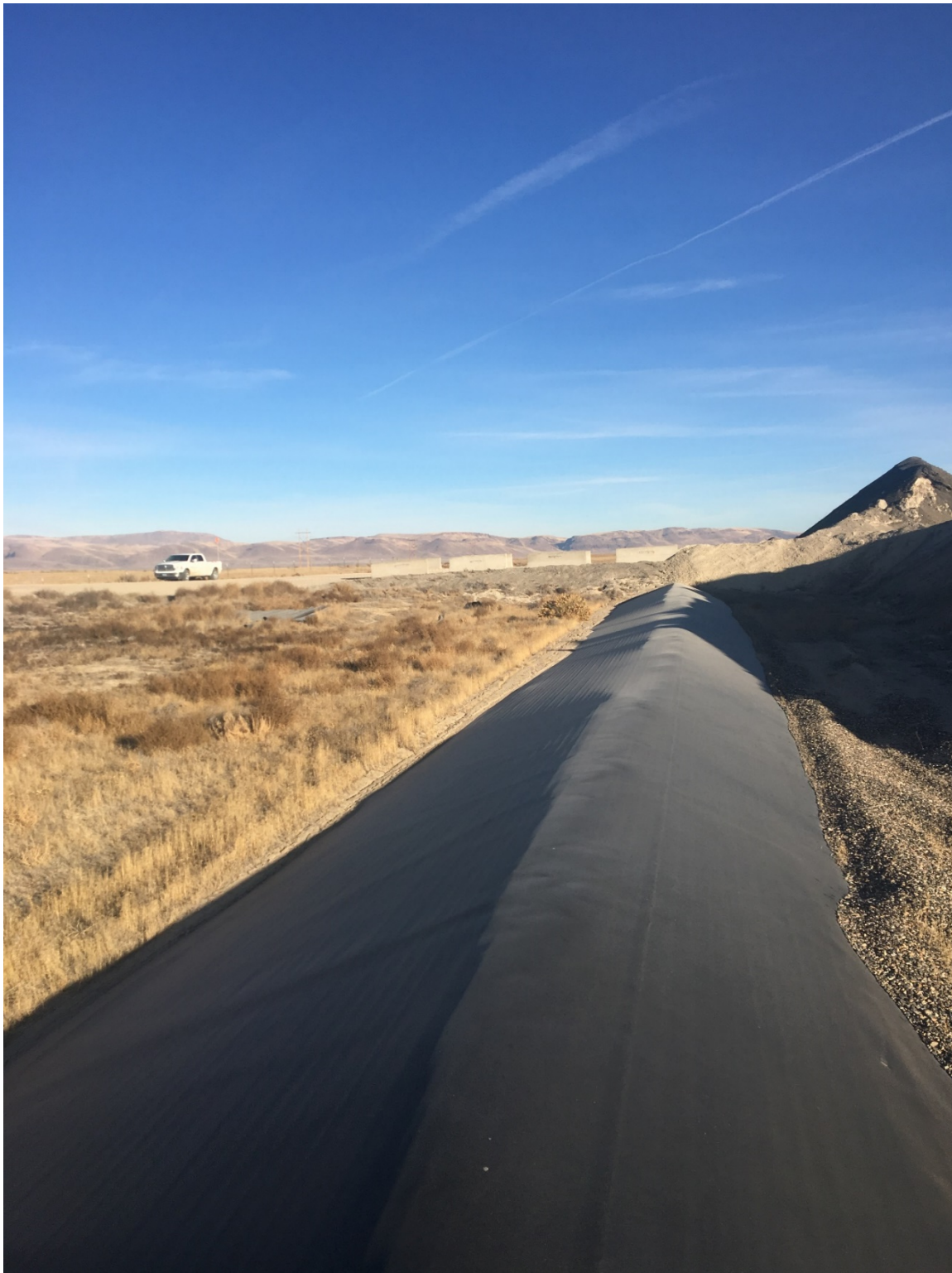
Photo 12. North Perimeter Berm, Southwest Corner, Cell 1 - View North
