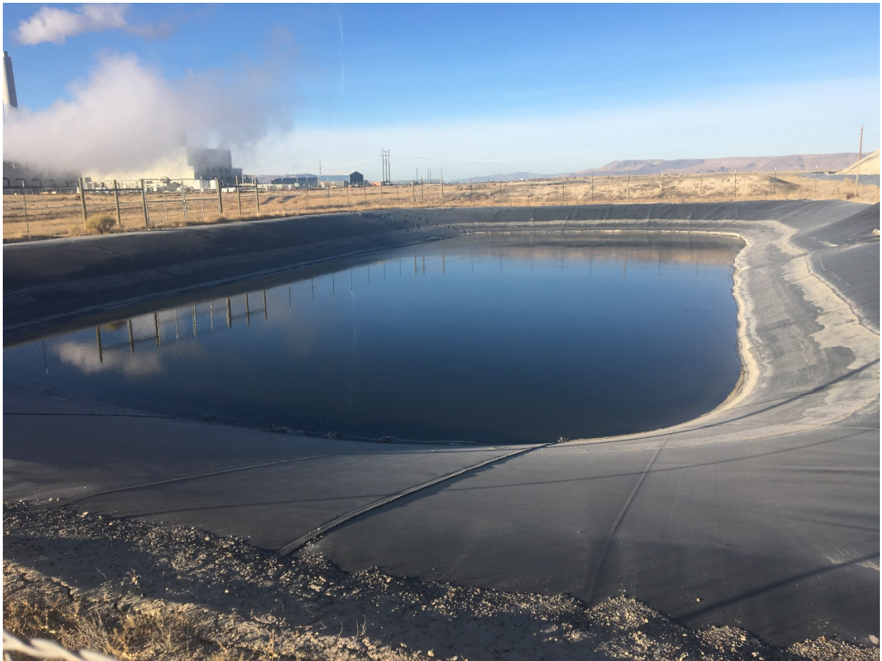
Photo 3. Collection Pond 1 - View West
