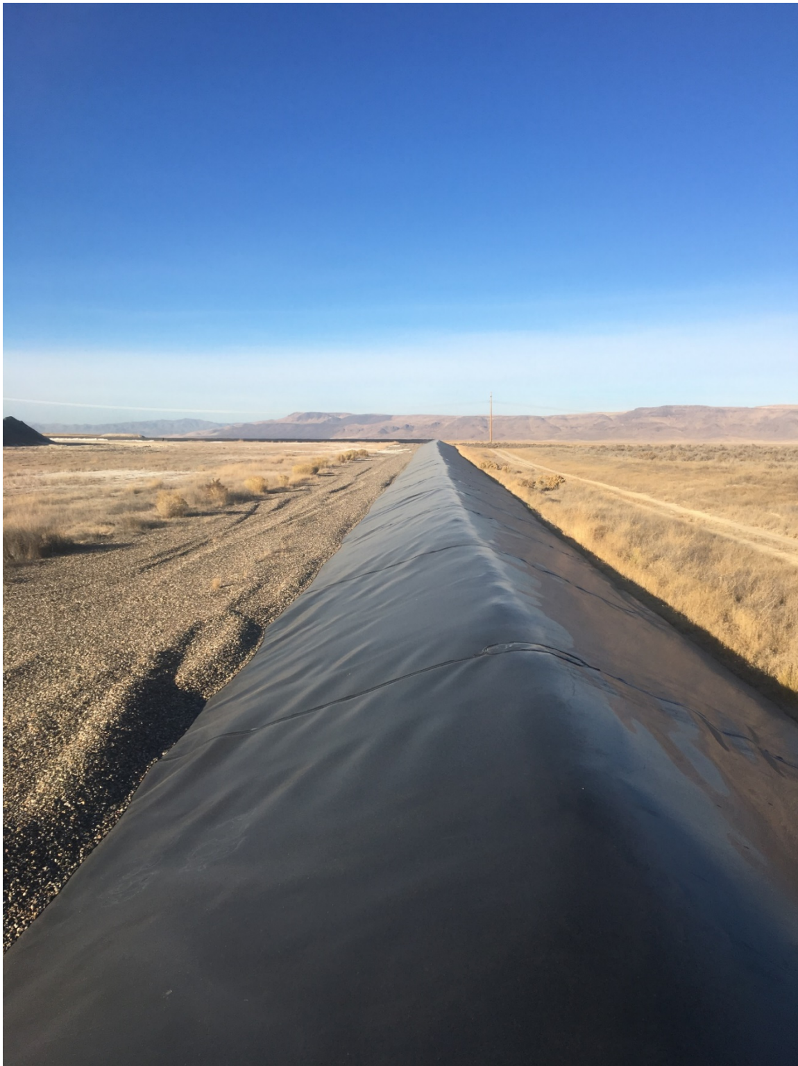
Photo 8. North Perimeter Berm, Northeast Corner, Cell 2 - View West
