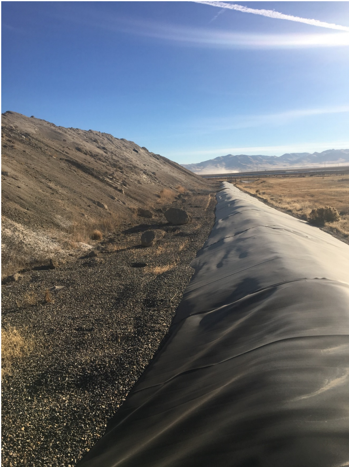
Photo 13. South Perimeter Berm, Southeast Corner, Cell 1 - View East
