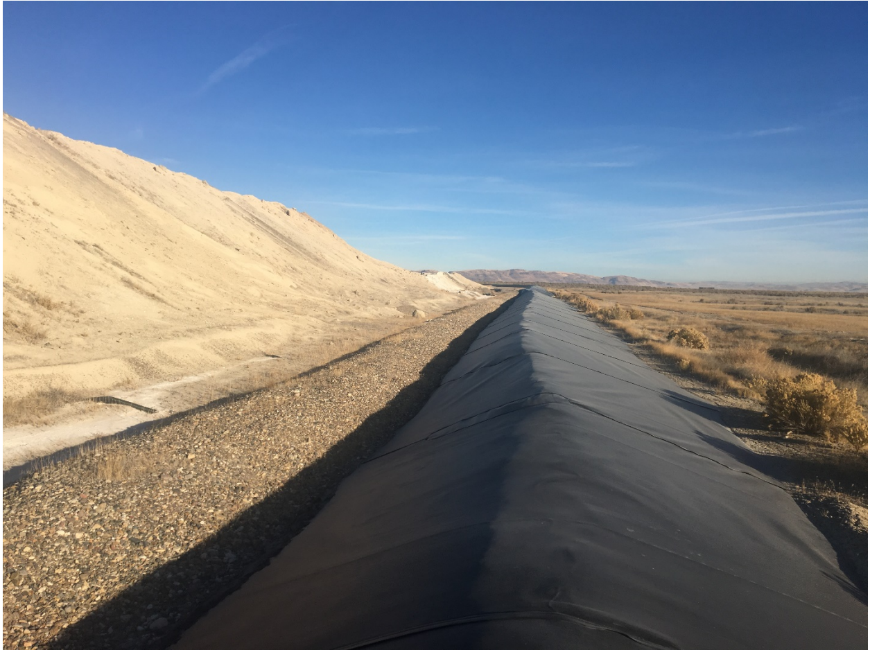
Photo 5. East Perimeter Berm, Southeast Corner, Cell 1 - View North
