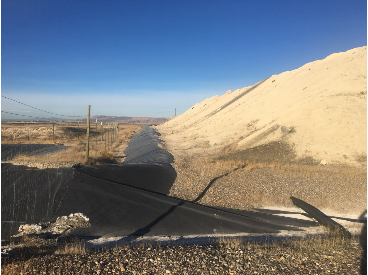
Photo 4. South Perimeter Berm, Southeast Corner, Cell 1 - View West
