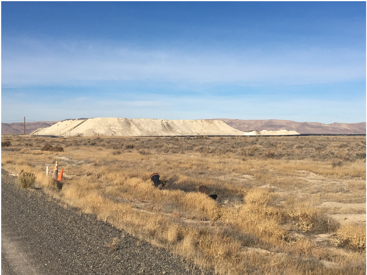
Photo 16. CCR Stockpile, Cell 1 and 2 - View West
