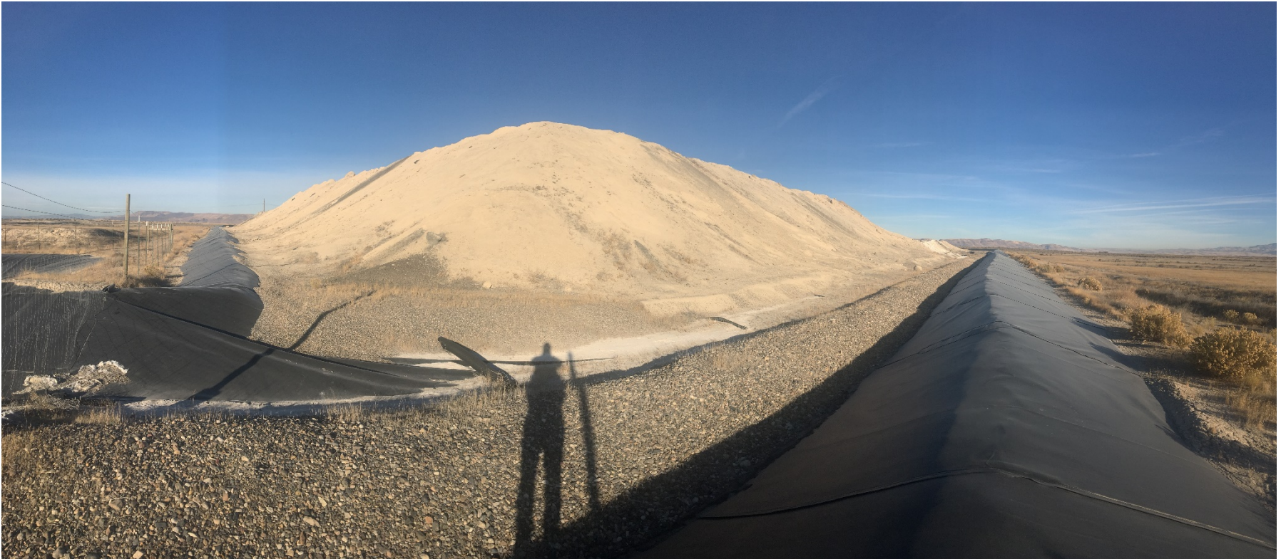
Photo 6. Southeast Corner of CCR, Cell 1 - View Northwest
