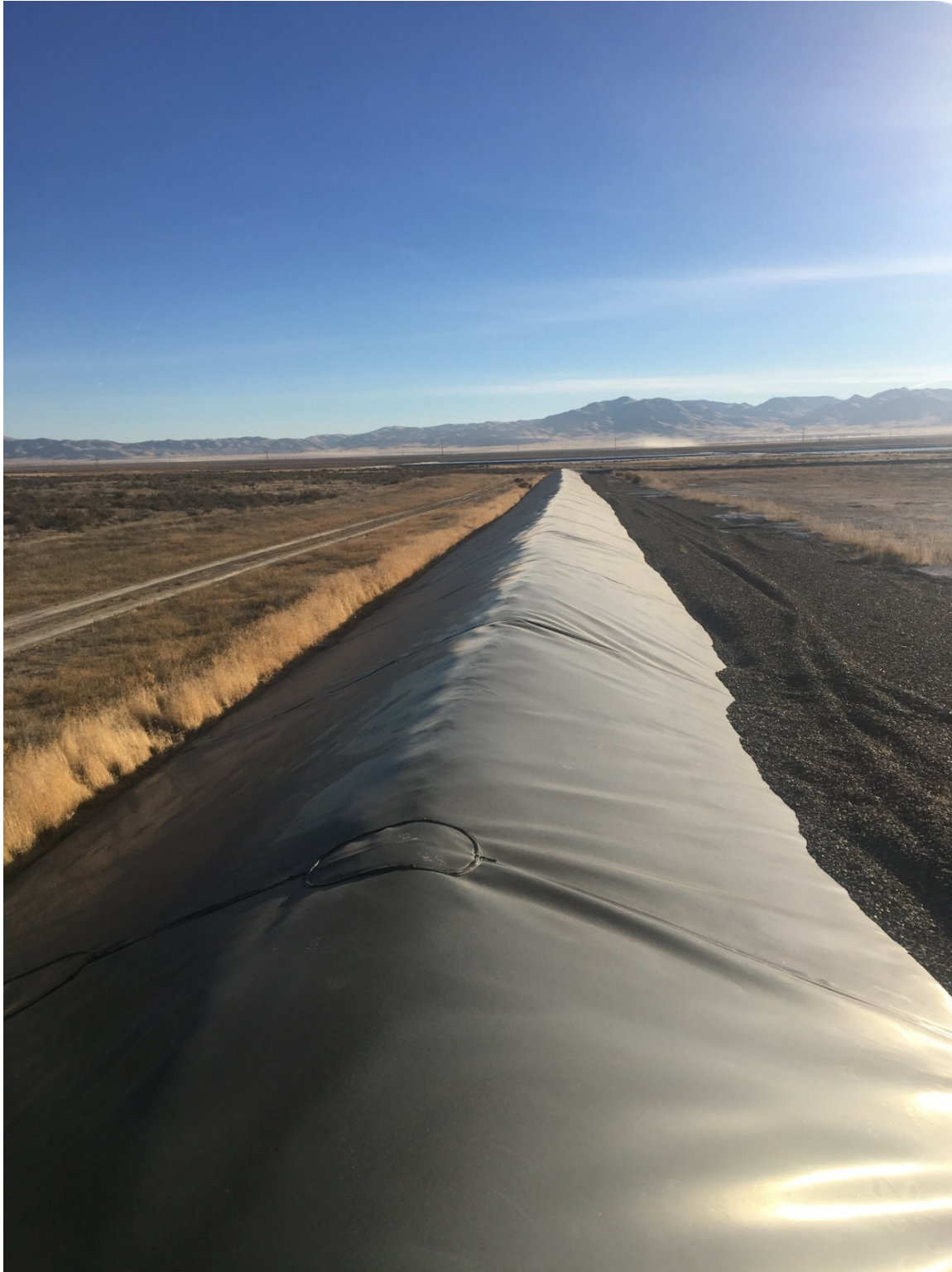
Photo 10. North Perimeter Berm, Northwest Corner, Cell 2 - View East
