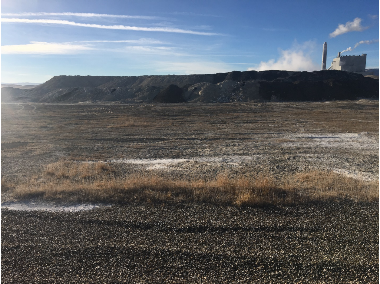
Photo 15. Cell 2 Deposition - View South
